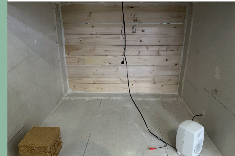
Provisional acoustic testing setup. Illustration: Grape architects
